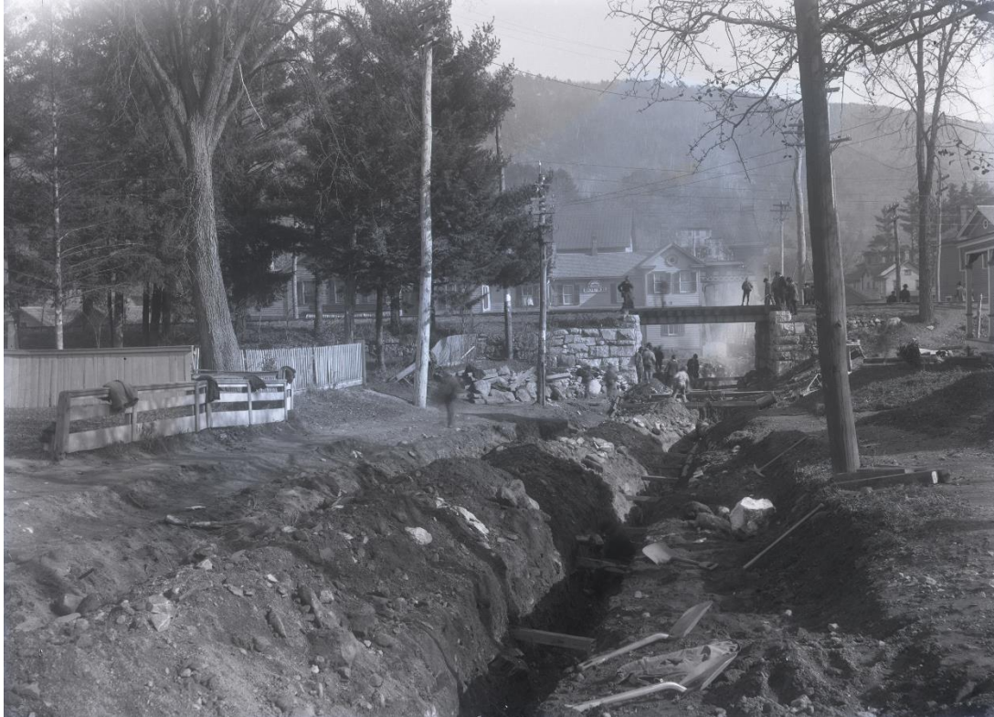
Cast Iron Main Installation on Pleasant Street circa 1900
